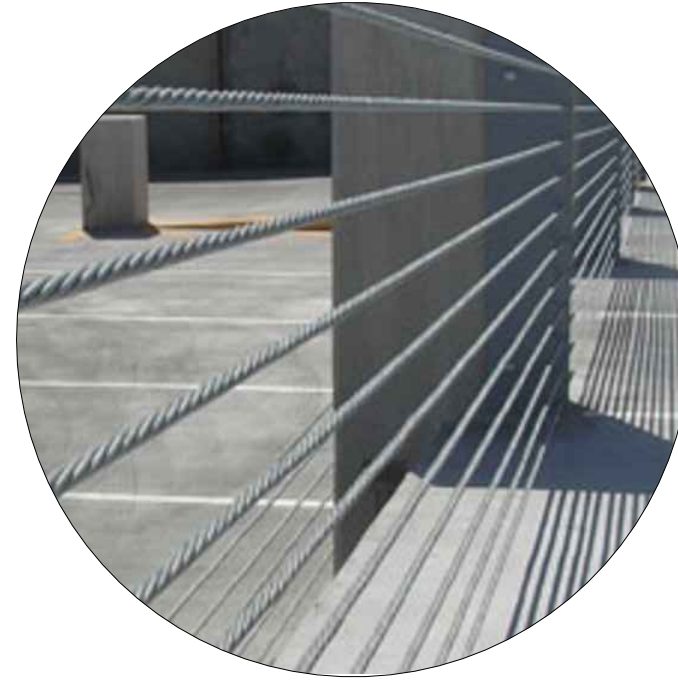
7 42" H. CABLE CRASH WALL (HORIZONTAL WIRES) SHOP DRAWINGS TO BE APPROVED PRIOR TO INSTALLATION
